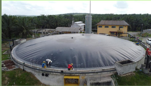
Anaerobic digesters
